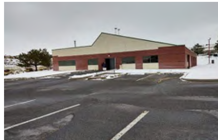
Figure 8 Business Technology Site lighting, Pole Light and Wall Pack
