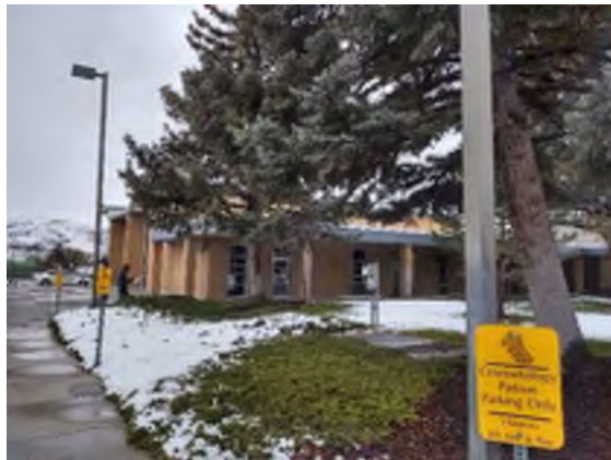
Figure 1 RFC Electrical Utility Vault
