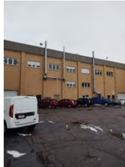
Figure 7 RFC Parking Lot Lighting Mounted on Roof
