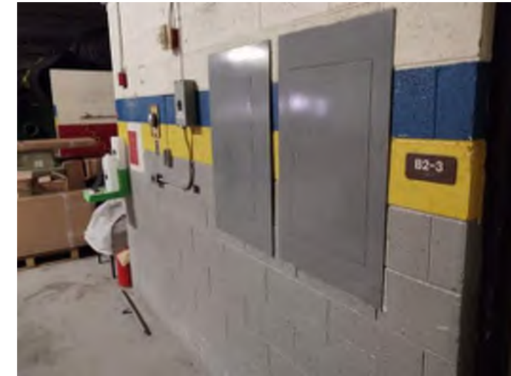
Figure 6 RFC South Recessed Panels, typical of panels in RFC.
